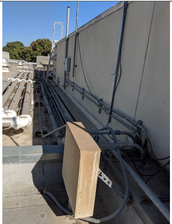
Photo of an electrical junction box on the roof. The electrical conduit extends to serve load in Building 940 and the admin building.
