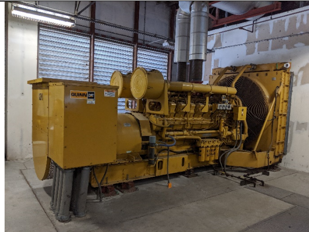
Photo of existing 2187 KW/ 1750 KVA generator.
