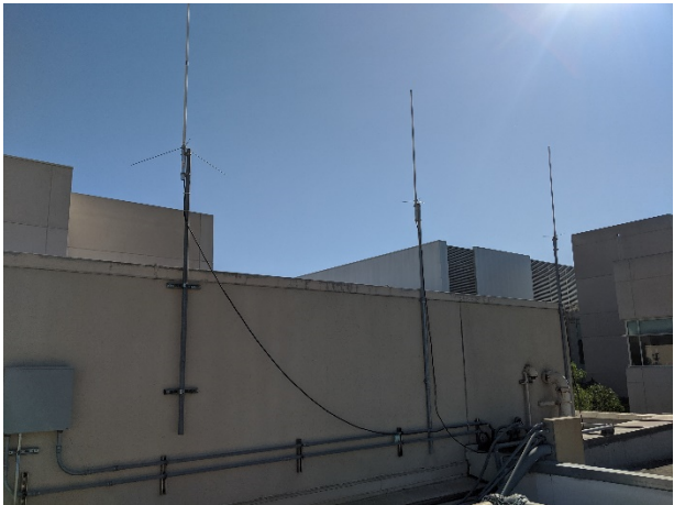
Photo of distributed antennae system on the roof.
