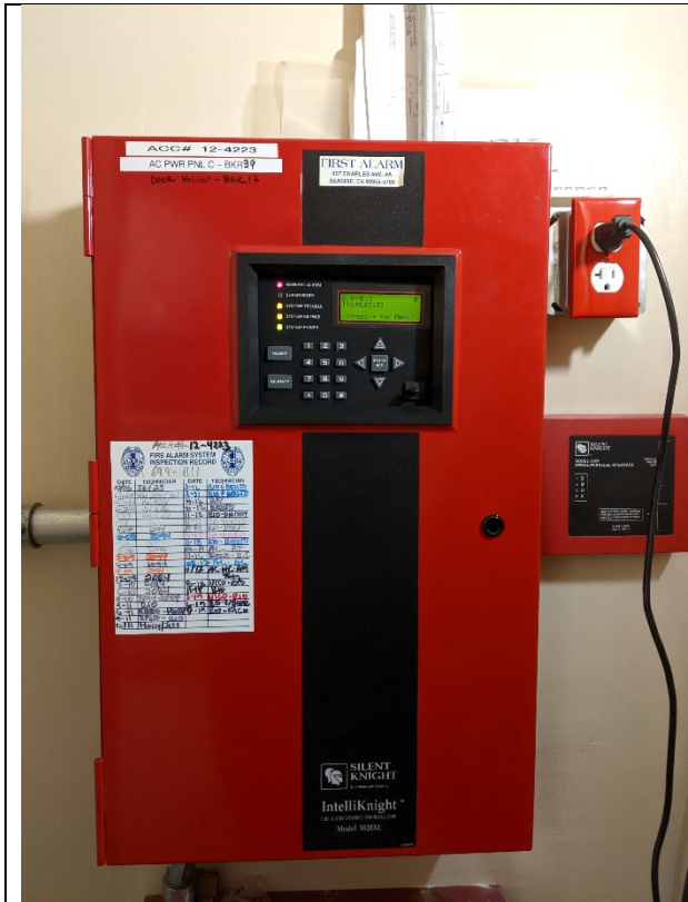
Photo of fire alarm panel connected to Panel C which is normal power.
